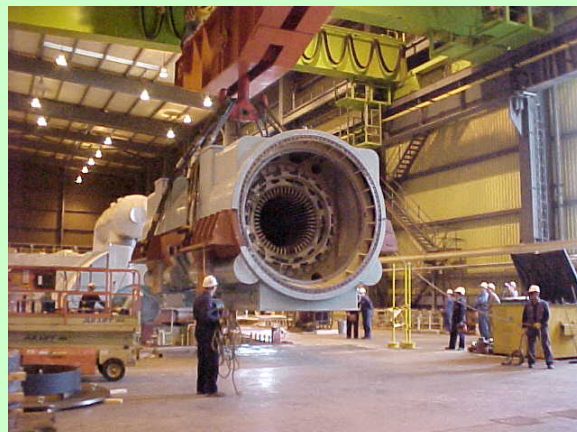
Rebuilding of 500MW Generator at Loy Yang 'B' Power Station
