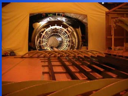
Tarong P.S. Unit 2 Generator Stator Rewinding
