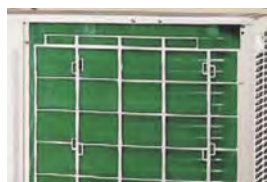
Green anti-corrosion coating pictured.
