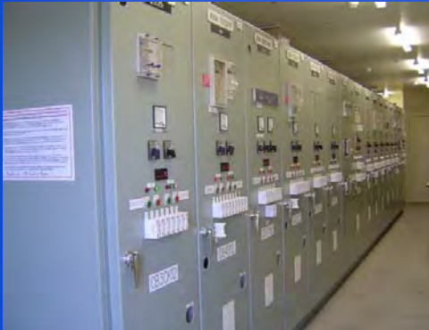
36kV Indoor Compact-GIS for Energex Ltd
