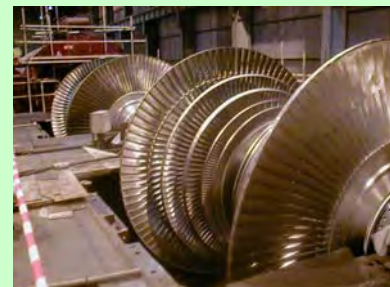
Liddell P.S. 500MW LP Turbine Upgrade
