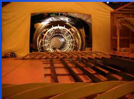
Tarong P.S. Unit 2 Generator Stator Rewinding
